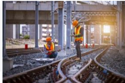
Infrastructure Condition Assessment
