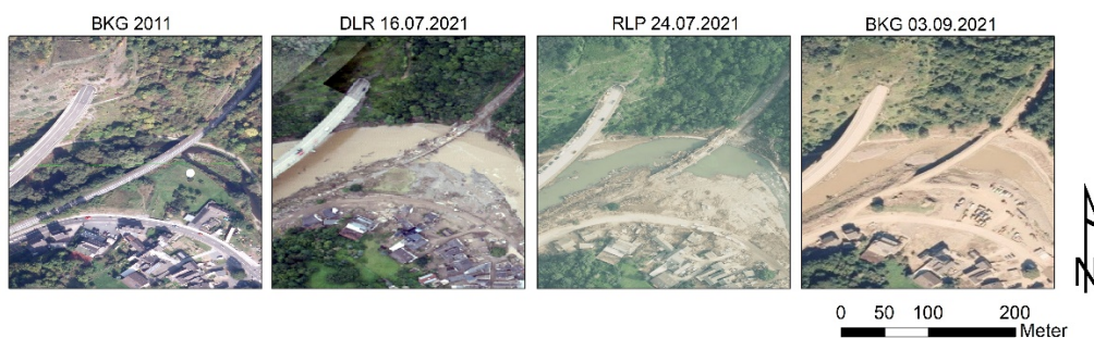
Figure 3. An example from the three different aerial photographs [37–39] showing bridge 3. The photograph from 2011 was taken as reference for the conditions before the 2021 event [40].
